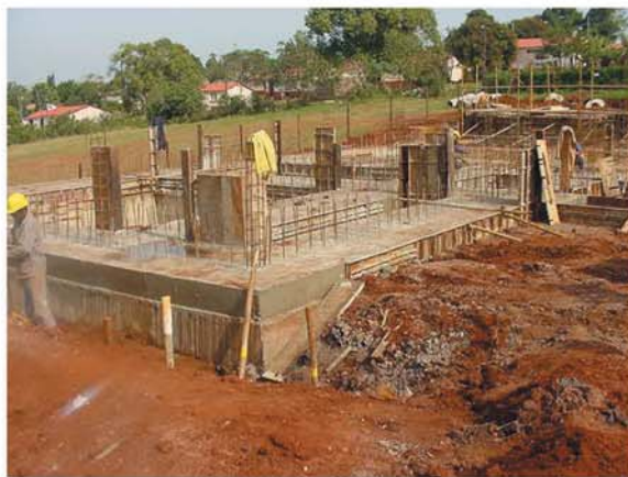
Construction of the Nsenleni Community Health Centre
