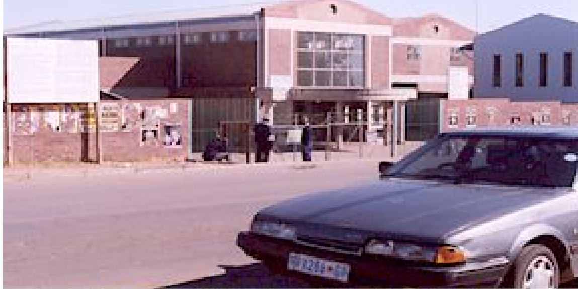
Charles Johnson Memorial Hospital
