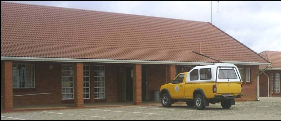
FRONT entrance of Nocomboshe Clinic. This clinic is situated in Umsinga Top approximately 25 km from Tugela Ferry. The area is so beautiful with its mountain and evergreen trees. It is under iNkosi Ngubane and it serves the community of Nocomboshe and surrounding areas.
