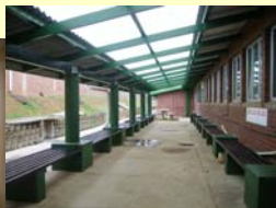
A sheltered waiting area was built after complaints from the community about unfavorable exposures to bad weather conditions.
