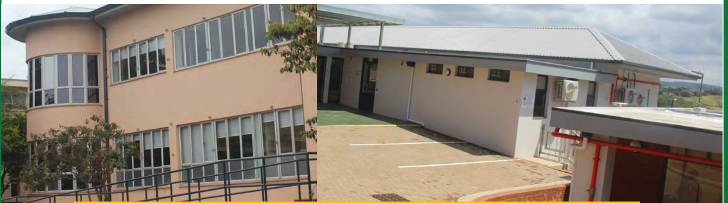
Newly Renovated 84 Bed Covid-19 Isolation Wards Officially Opened by MEC for Health KZN
