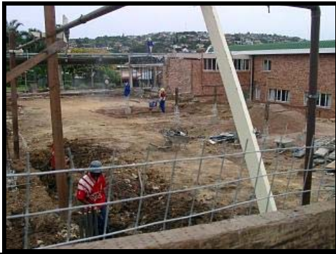
Construction underway for the new paediatrics
