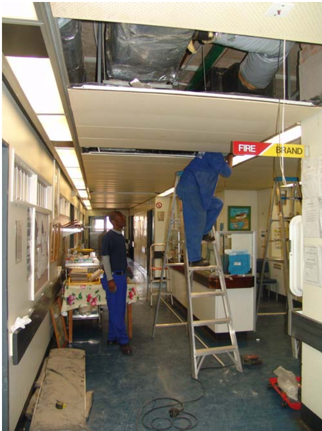
Fire detection systems are being installed throughout the hospital.
