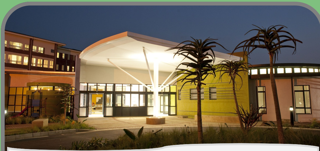
Night view of the new building– BHP Billiton Paediatric Centre of Excellence
