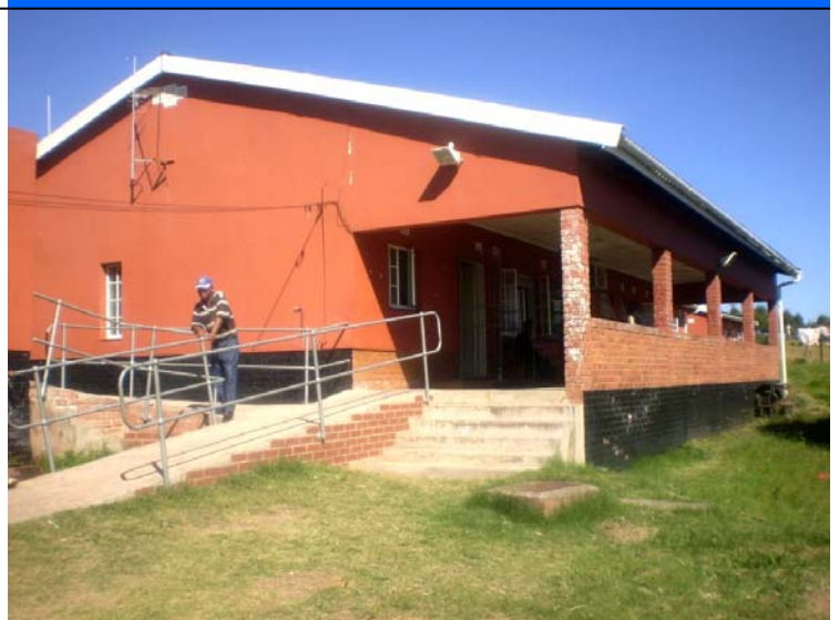
Renovations at Zwelibomvu Clinic
