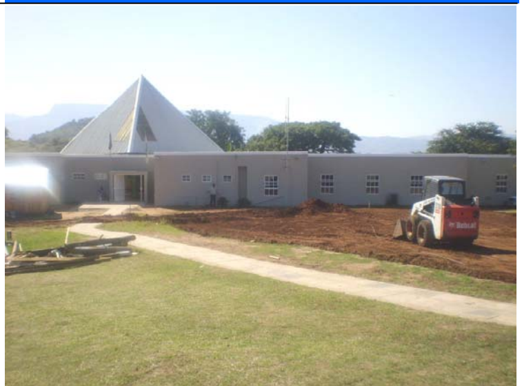
Refurbishment at Ngcolosi Clinic
