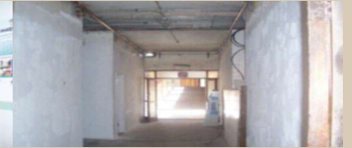
Pharmacy waiting area - during the latest renovations
