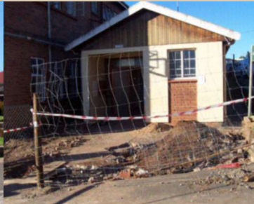
Main entrance (during renovations)
