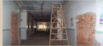
Pharmacy waiting area - at the beginning of renovations
