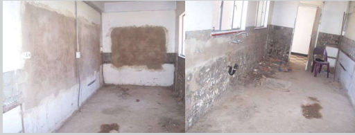
Before (the staff residence kitchen)
