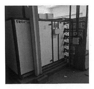
This system is in good condition and it runs with 407c gas, during our investigation we discovered that units tripped on low gas which then we pressure tested the systems discovered gas leaks on suctions and discharge ports, closed those valves accordingly than regased units and switch them off. Because unit and room must be pressure cleaned first before usage for hygiene purposes
