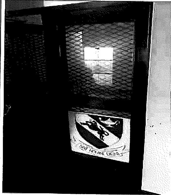
Image No. 7: Install custom made retractable sliding gates fabricated from powder coated hot dipped galvanized mild steel as per the Department of Health's colour choice as per the manufacture's specification. at main exit points
