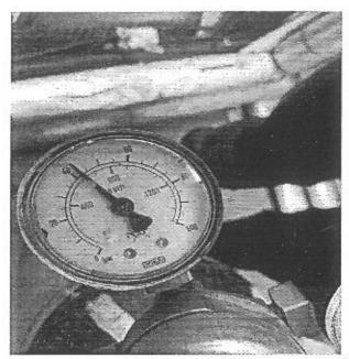
Pressure tested chiller 1 system to 43 bars and discovered few leaks in the system, the leaks were discovered on the liquid line drier that's why we recommend it must be replaced as well as Schrader valves. Once all leaks are repaired system must be pressure tested than the system will be ready for evacuation, re-gassed and commissioned.
