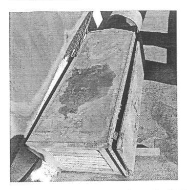
Fresh air fan, paint the panel with galvanised paint or silver paint then replace filter as per existing one and make sure fan is running, also repair those hinges so that cover will close properly.
