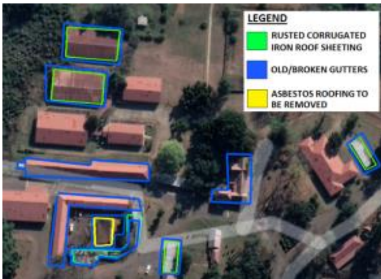
Figure 3: Site findings at the workshop offices, storage facilities adjacent facilities
