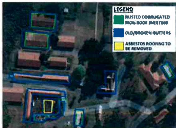
Figure 4-3: Site findings at the workshop offices, storage facilities adjacent facilities
