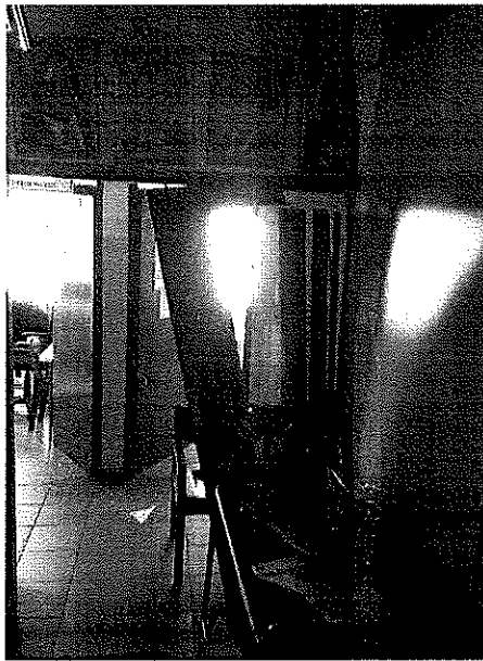
Block A- patient files room double entrance door broken, frame loose from wall
