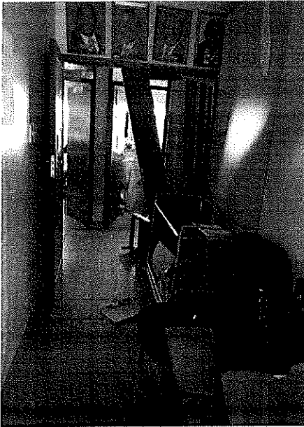
Block A- patient files room double entrance door broken, frame loose from wall
