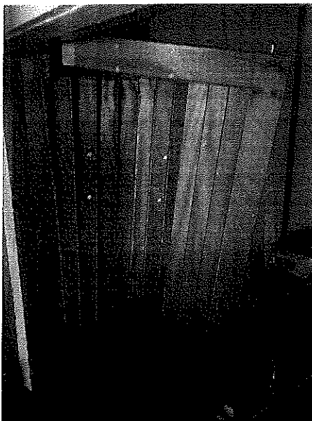
Block A- patient files room double entrance door broken, frame loose from wall
