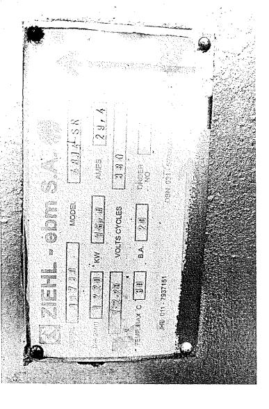
BILL OF QUANTITIES: FOR Regional Laundry Cato Manor Replace motors (x2) **SERVICE: ZNQ NUMBER: CONTRACTOR NAME CONTACT PERSON CONTACT DETAILS** ITEM UNIT **AMOUNT** DESCRIPTION QTY RATE **CODE**: Replace motors Remove damaged motorsfbr Each 2 Supply, deliver and install 15Kw motors and ensure that the motors are operating 2 Each 2 perfectly .Attached is the name plate of the old motor **SUB TOTAL** VAT TOTAL
