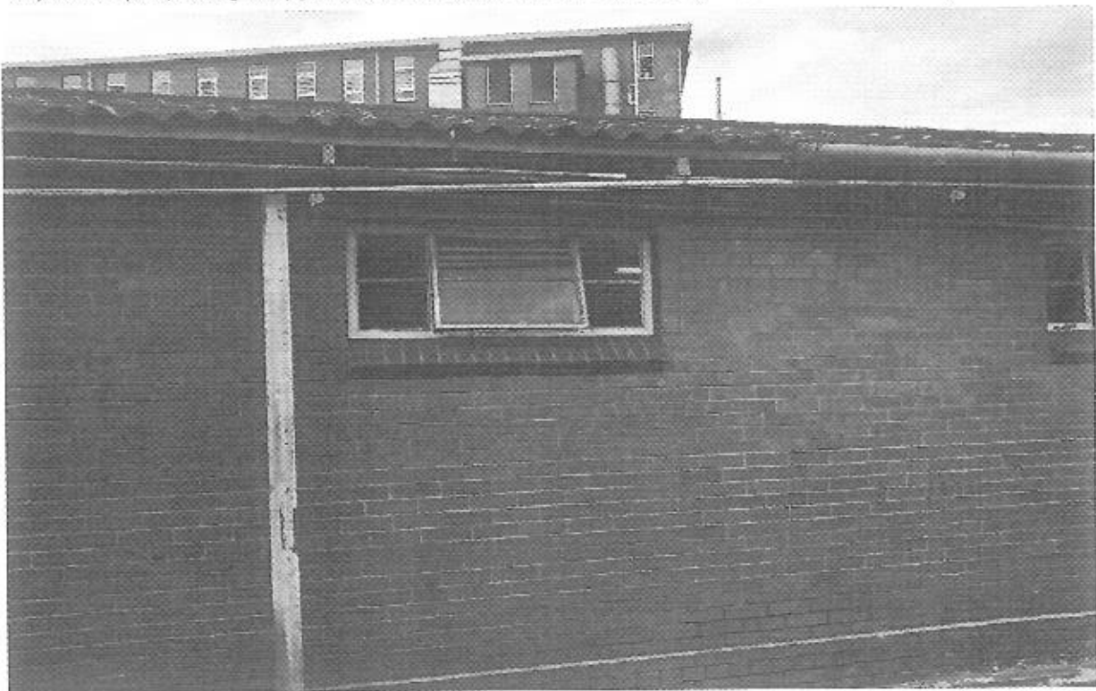
Physiotherapist passage oxygen line hanging out need to be properly mounted & color coding.
