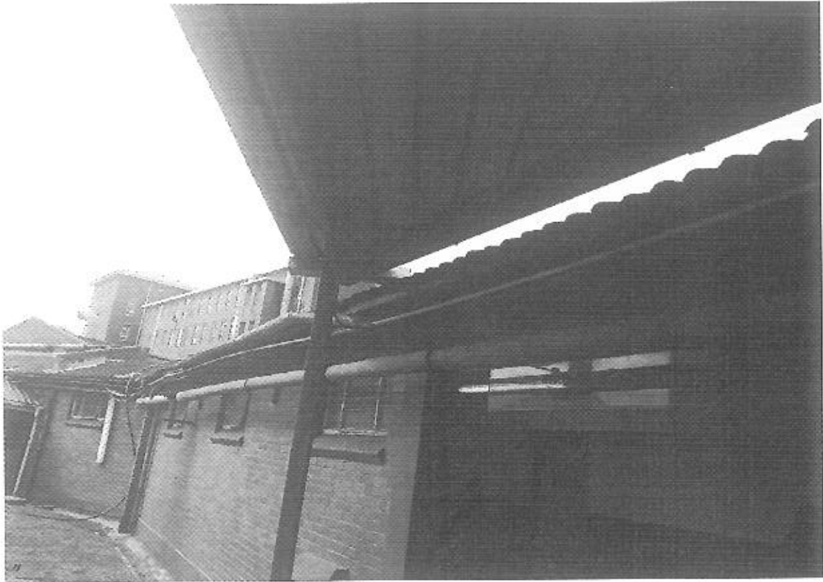
Physiotherapist passage oxygen line hanging out need to be properly mounted & color coding.
