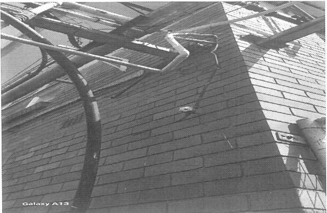
Color coding and replace bended pipeline.
