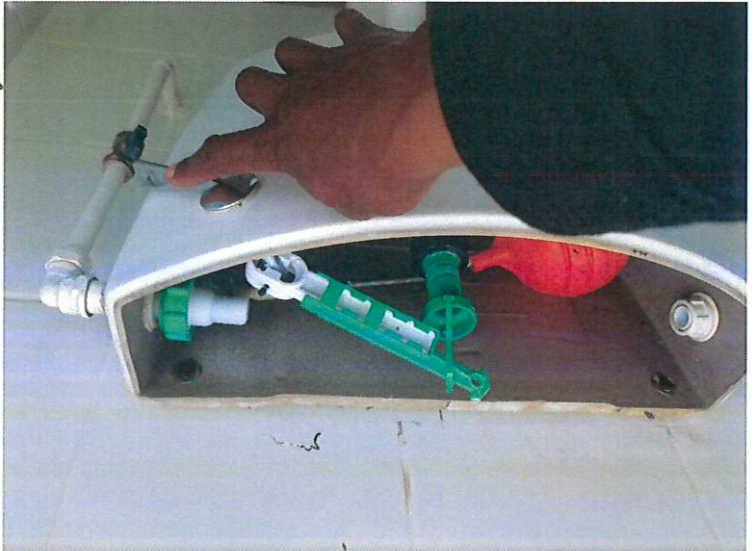
Water Inlets Toilet 30 Ball Valve (side view)
