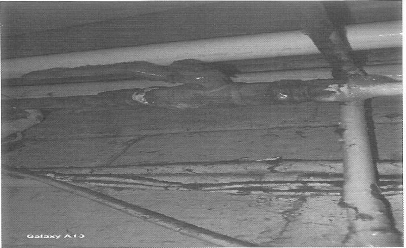
Old building main line cutted off, leaking need to be properly closed see attached pictures.
