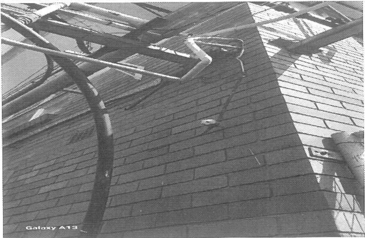
Color coding and replace bended pipeline.
