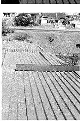
**FINDINGS**: 7 x Zincalume Barge boards blown off and damaged by wind.
