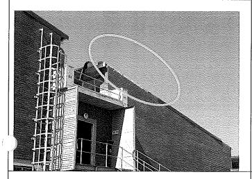
**FINDINGS**: 24 x Zincalume Barge boards blown off and damaged by wind.
