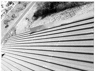
**FINDINGS**: 24 x Zincalume Barge boards blown off and damaged by wind.
