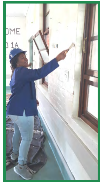
Sister Khumalo scrapping the wall before it can be painted
