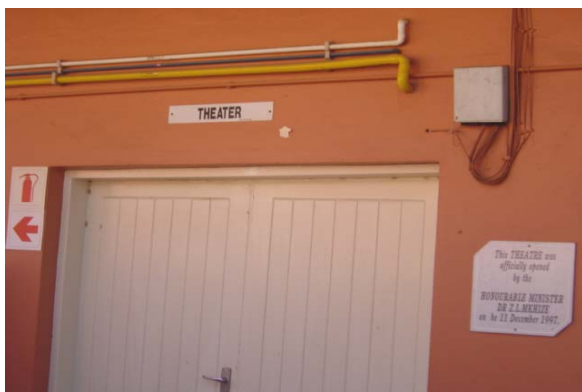
OPERATING THEATRE BEFORE
