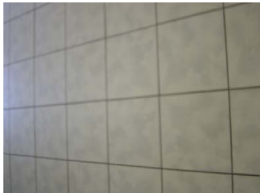
VCT FLOORS AFTER
