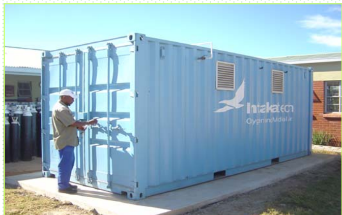
New Hospital gas bank recently install for oxygen gas generation to minimize renting and high ordering of oxygen gas cylinders, this initiative is going to relieve cost burden on the Hospital budget.
