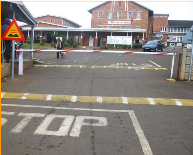
Speed humps at the entrance of the Hospital
