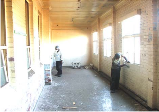
Contractors hard at work with renovations
