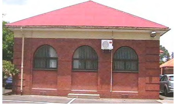
2008 Admin verandah converted to HR offices
