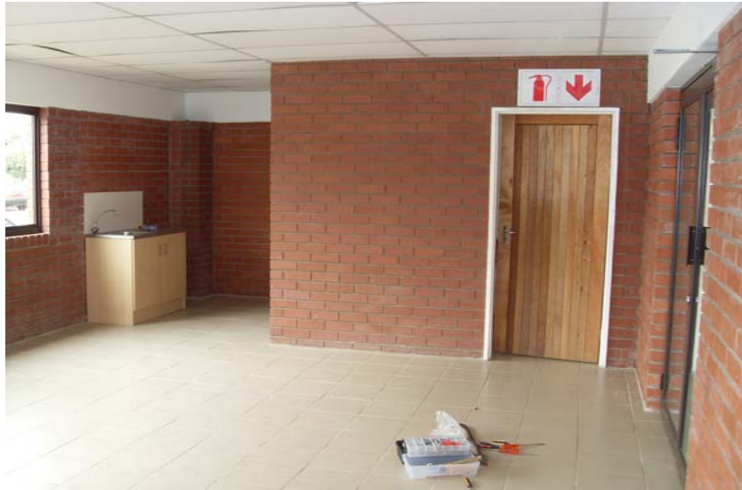
Conversion in progress
