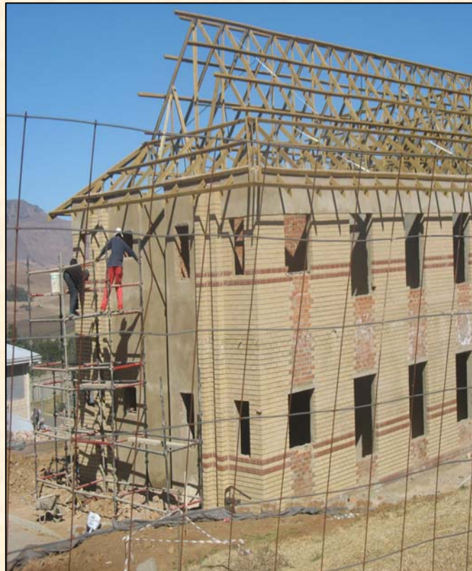
Construction workers busy working on the new nurses home
