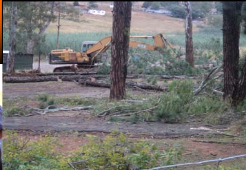
NEW OPD IN PROGRESS
