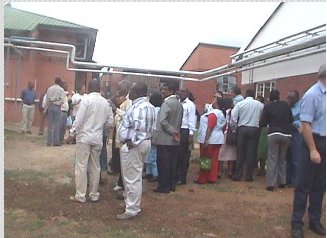
The Delegates checking the renovations of Male ward soon to be TB ward.
