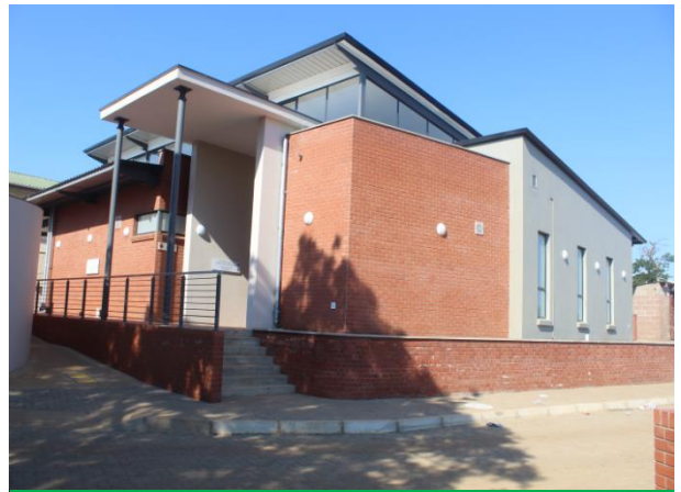
Newly Completed Health Allied Building temporarily to house OPD
