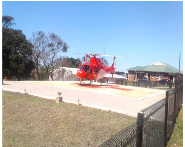
Helipad is now in use as well as the renovated Male Ward
