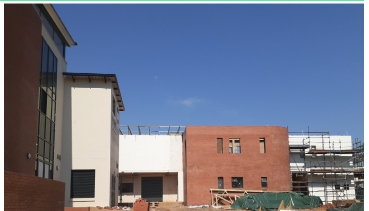
Side view of new OPD (Pharmacy bulk stores receiving )
