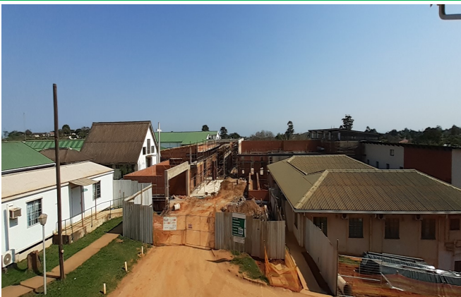
Back view of the OPD (Trauma unit) under construction.
