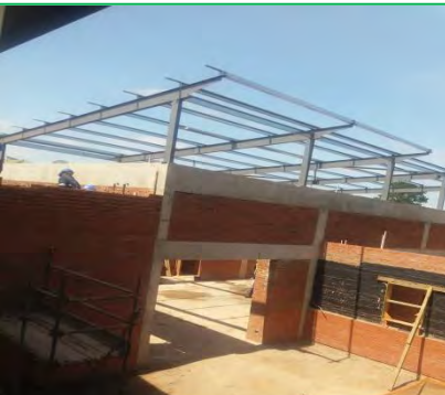
Construction of Allied Health Service Building at Hlabisa Hospital
