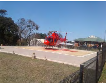
Helicopter comfortable in the newly build helipad at Hlabisa Hospital
