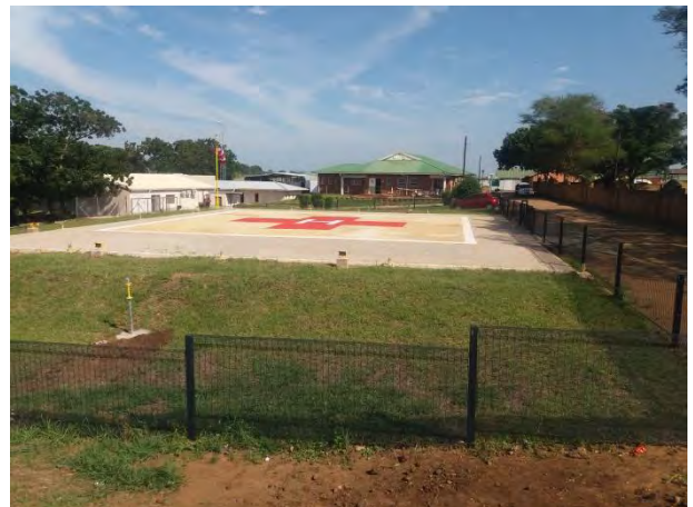
Newly built helipad that will ensure day and night air-lifting of patients
