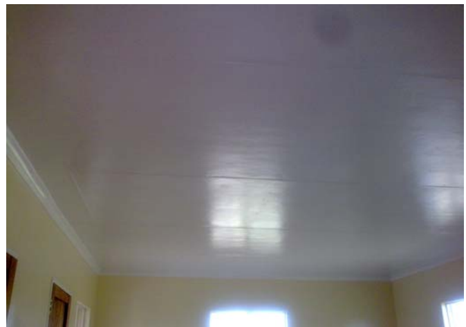
Inside Nsunduzane Clinic after renovations
