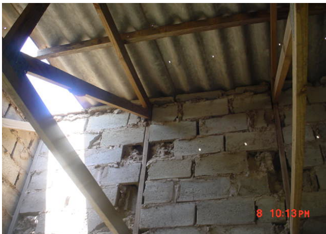
Inside Nsunduzane Clinic before renovations
