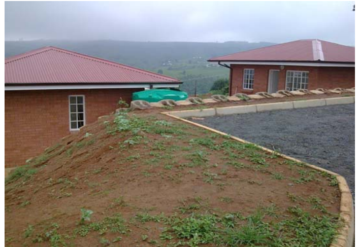
KwaNyuswa Clinic, residence and paving
