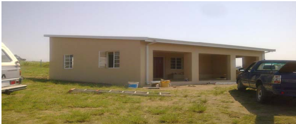
Nsunduzane Health Post after renovations
