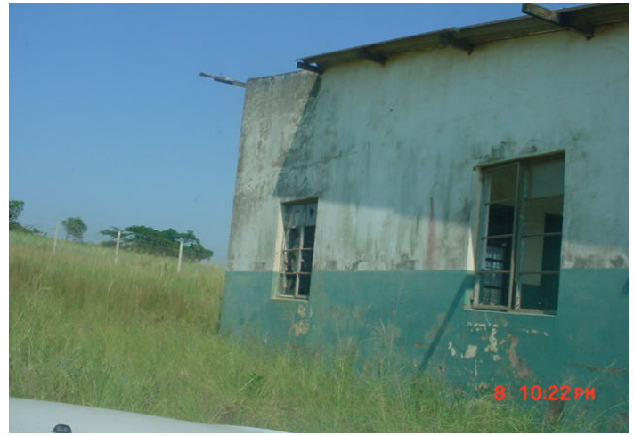
Nsunduzane Health post before renovations
