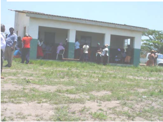
Nsunduzane Health Post before renovations
