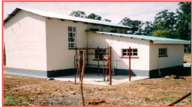
The Maintenance Building, which includes Workshop, artisan electrician ,plumbers etc.
