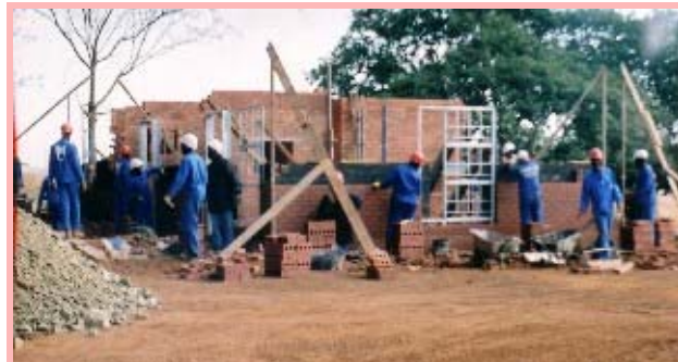
The new hospital structure for staff accommodation in process.
