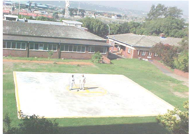
New Helipad situated opposite the Labour Ward
