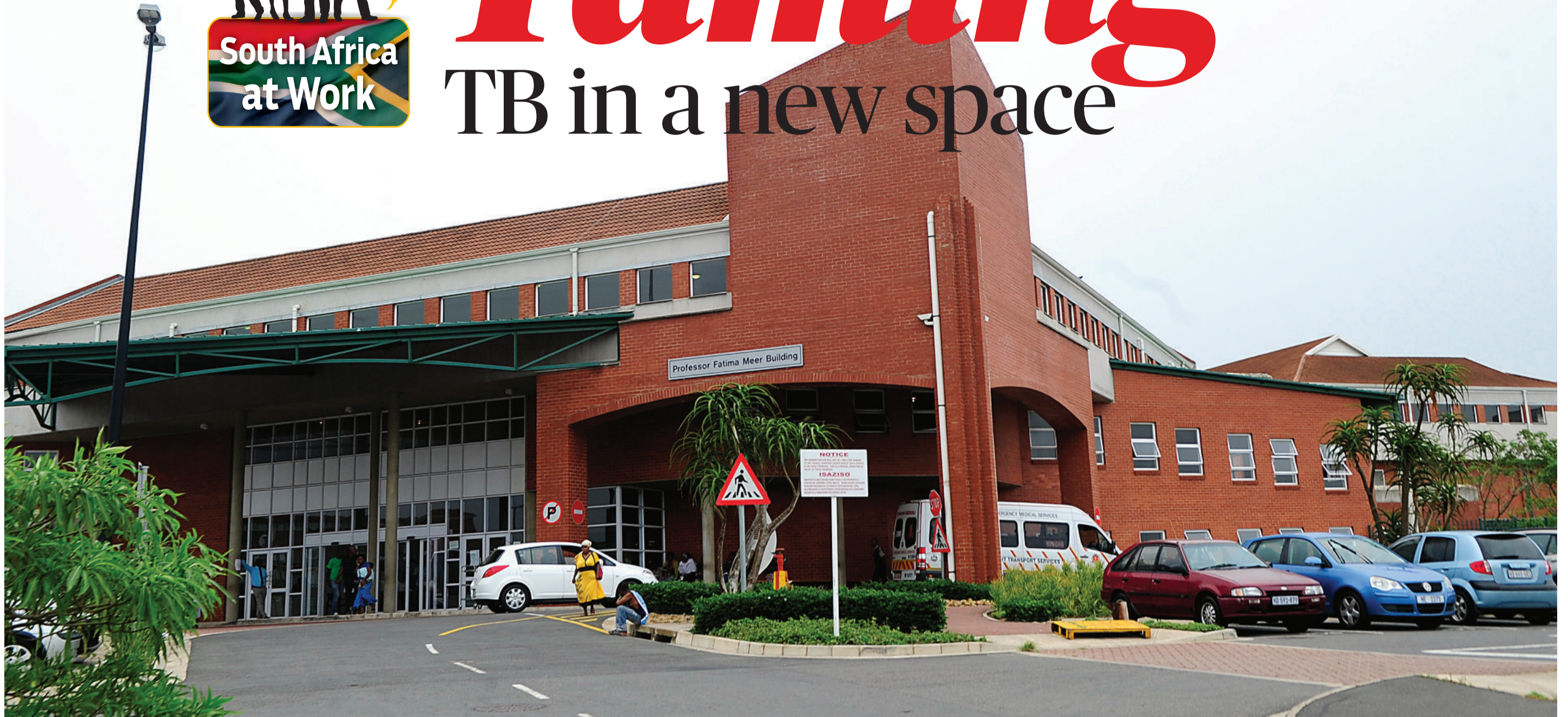
FACE-LIFT: King Dinuzulu Hospital has been completely overhauled, much to the delight of its staff members and patients
