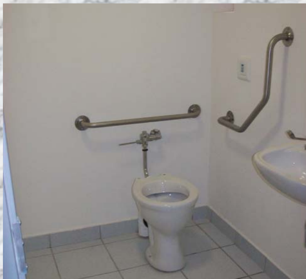
Ablution facility for disables people
