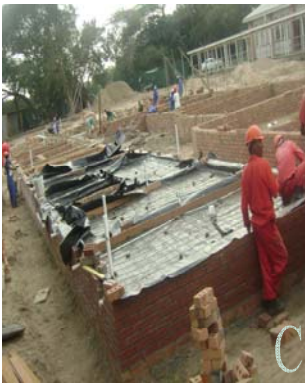
New pediatric ward on construction
