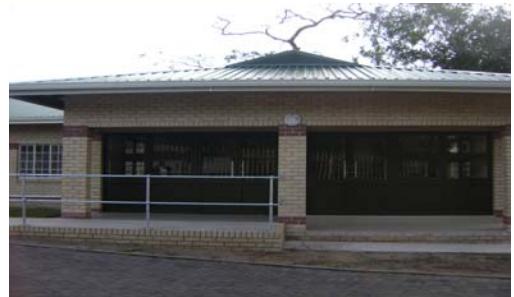
New PMTCT Block nearing completion
