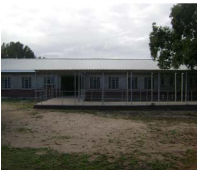
New pediatric ward on completion phase
