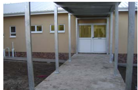
New isolation ward next to male ward nearing completion.
