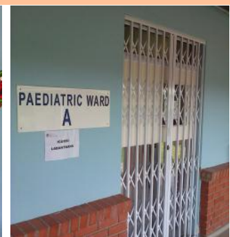
Installation of burglar guards in all wards
