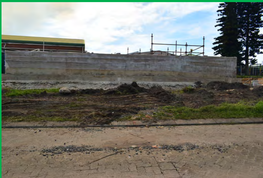
Water pipeline installation along OPD Pathway
