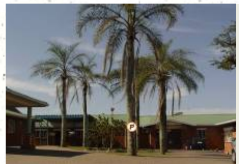
Front view of the hospital
