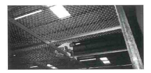
Suspended Ceiling Chain Link Wire Mesh
