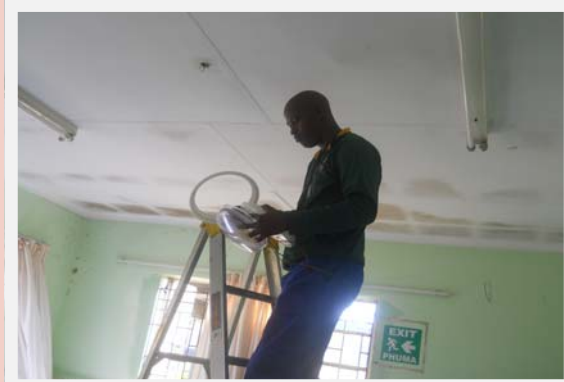
Mr. I. Z. Mazibuko– electrician fixing the globe
