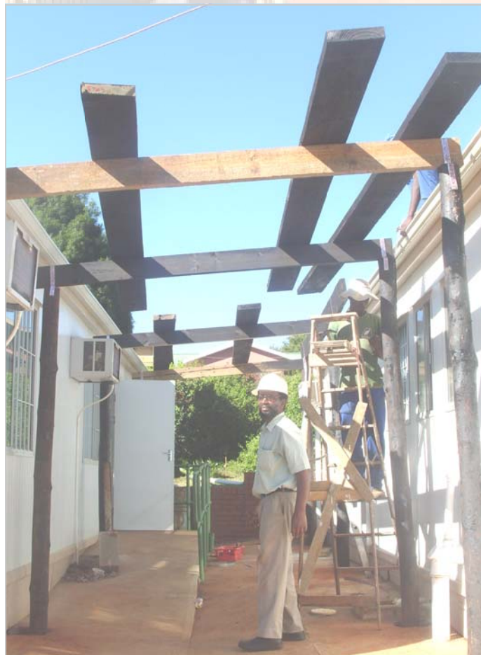
Adjacent: Construction of another shelter which will connect the two park-homes.
