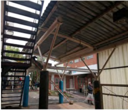
BEFORE—WAL-WAY TO NEW OPD SIDE SHEETING
