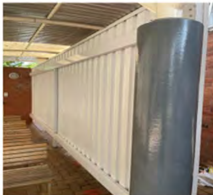
BEFORE—WAL-WAY TO NEW OPD SIDE SHEETING
