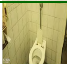
BEFORE—OPD PATIENT TOILET SYSTEM
